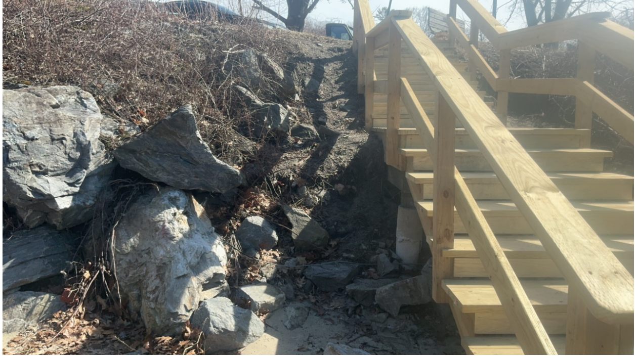
Figure 3: Photo of the new access stairs at Ferry Beach.
