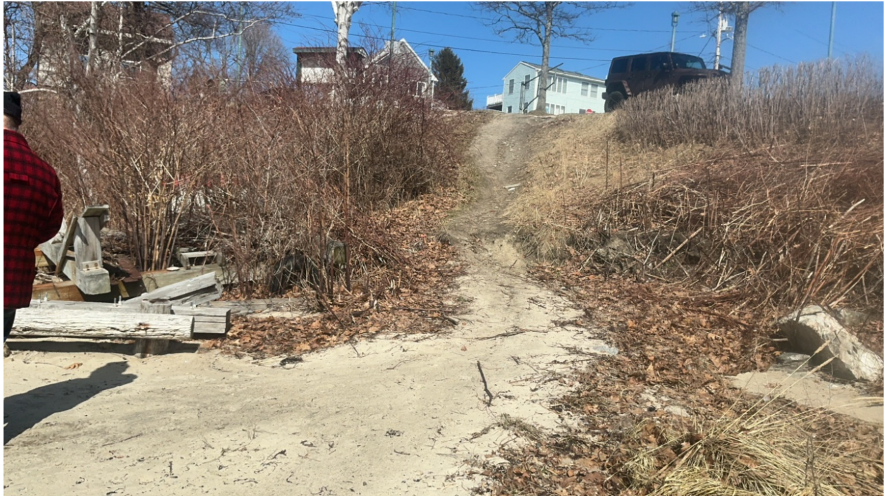
Figure 1: Photo of a section of the Ferry Beach bank including the footpath.
