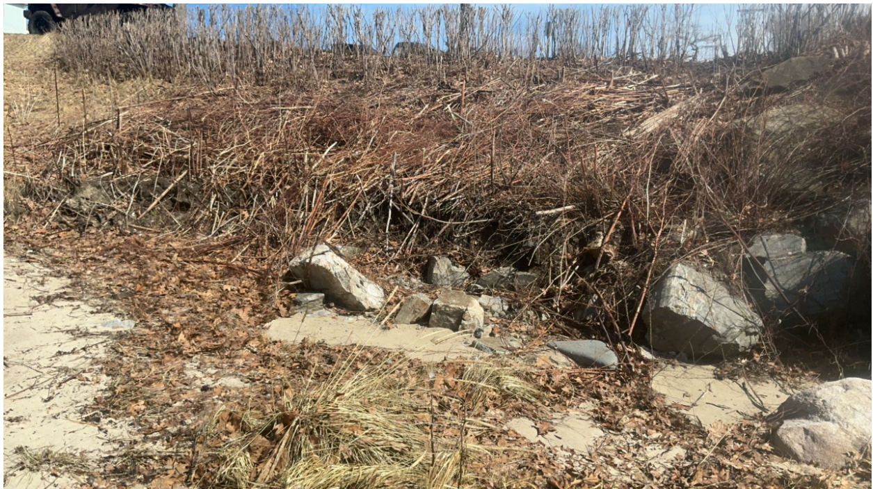
Figure 2: Photo of a section of the Ferry Beach bank between the footpath and access stairs.
