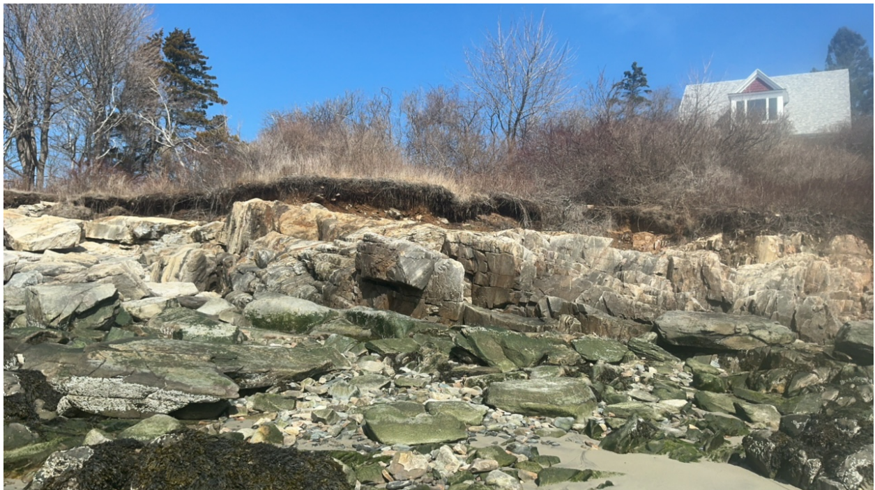
Figure 2: Photograph of the bank of the focus area of Sandy Beach. Undercutting of the soil layer above the bedrock is visible.
