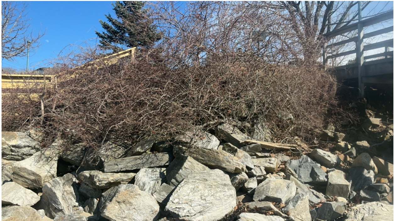
Figure 4: Photo of a section of the Ferry Beach bank between the access stairs and southern end, including the existing stone revetment.
