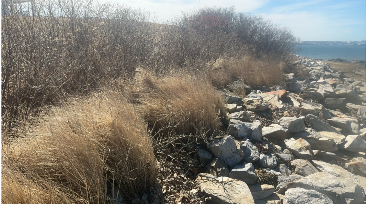
Figure 5: Photograph of existing riprap stabilization on a private property adjacent to the Centennial St boat ramp.
