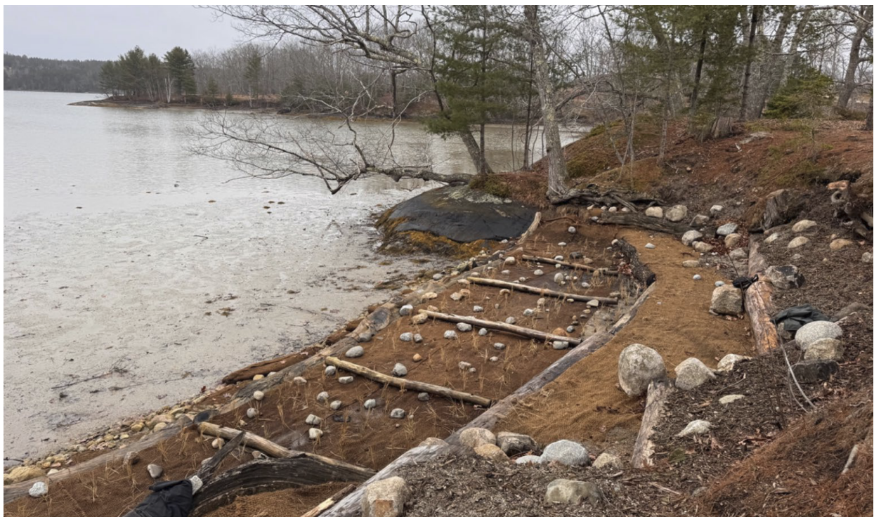
Figure 10: Example of a log sill installed for marsh restoration. (Photo from Treyball & Bernacki, 2025).
