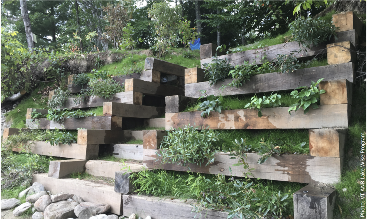
Figure 12: Example of a living crib wall from the Vermont Bioengineering Manual.
