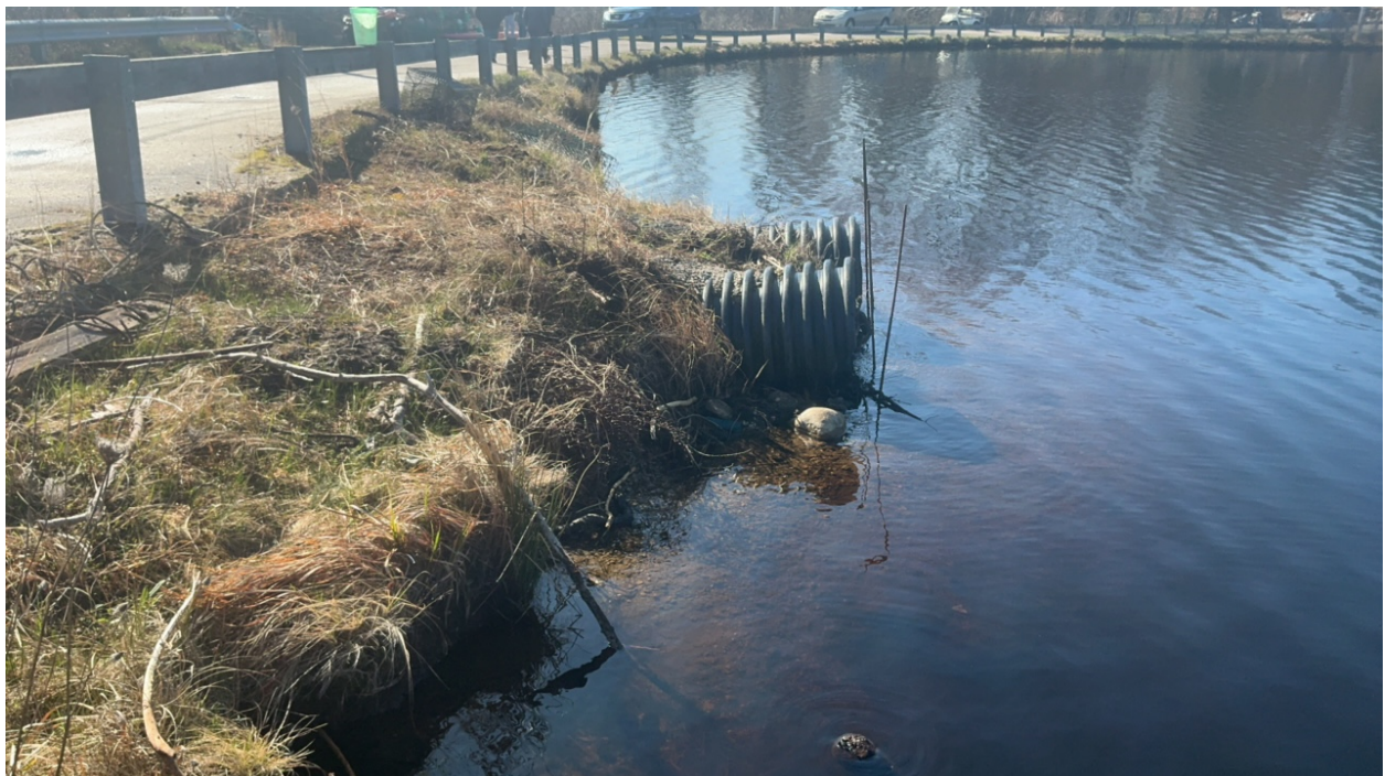
Figure 2: The shoreline of the freshwater pond and the inlets to the culvert underneath Fern Avenue.
