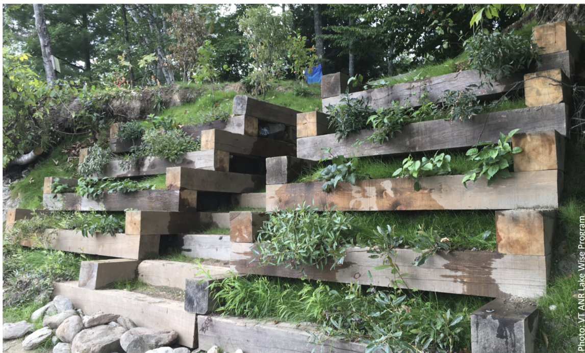
Figure 10: Example of a living crib wall from the Vermont Bioengineering Manual.
