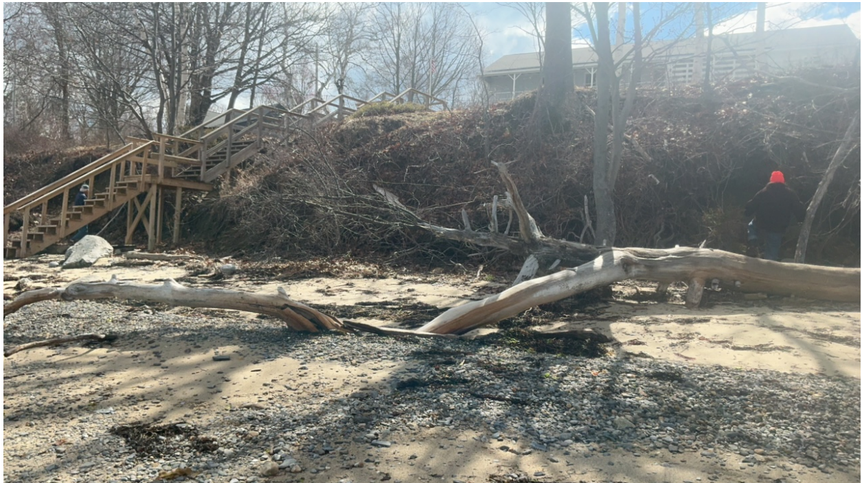
Figure 2: A section of the beach and coastal bluff at the VFW Hall including the shoreline access stairs.
