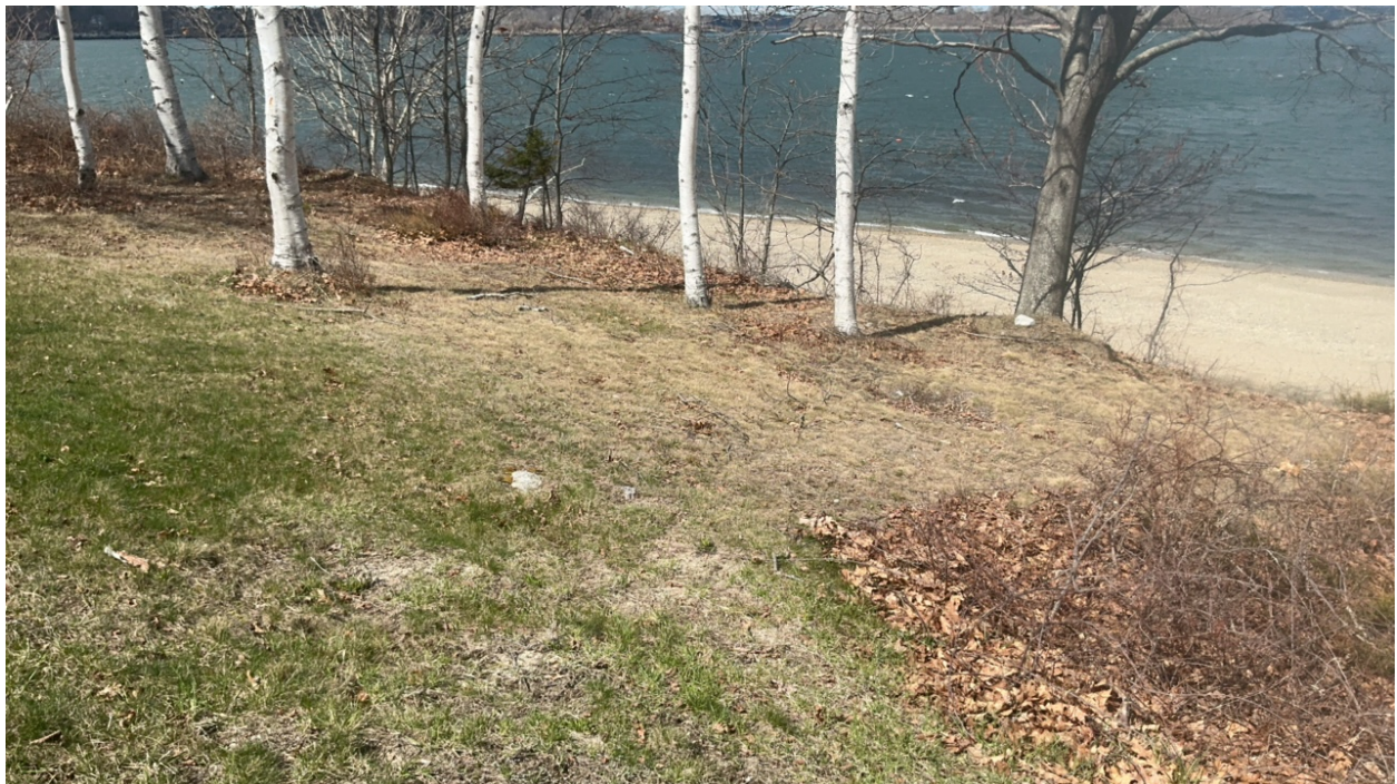
Figure 4: Bluff crest and upland areas at the VFW Hall.
