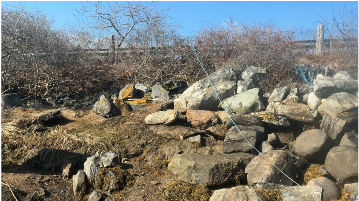
Figure 4: The tidal shoreline to the left of the culverts showing the transition from placed stones to salt marsh vegetation.
