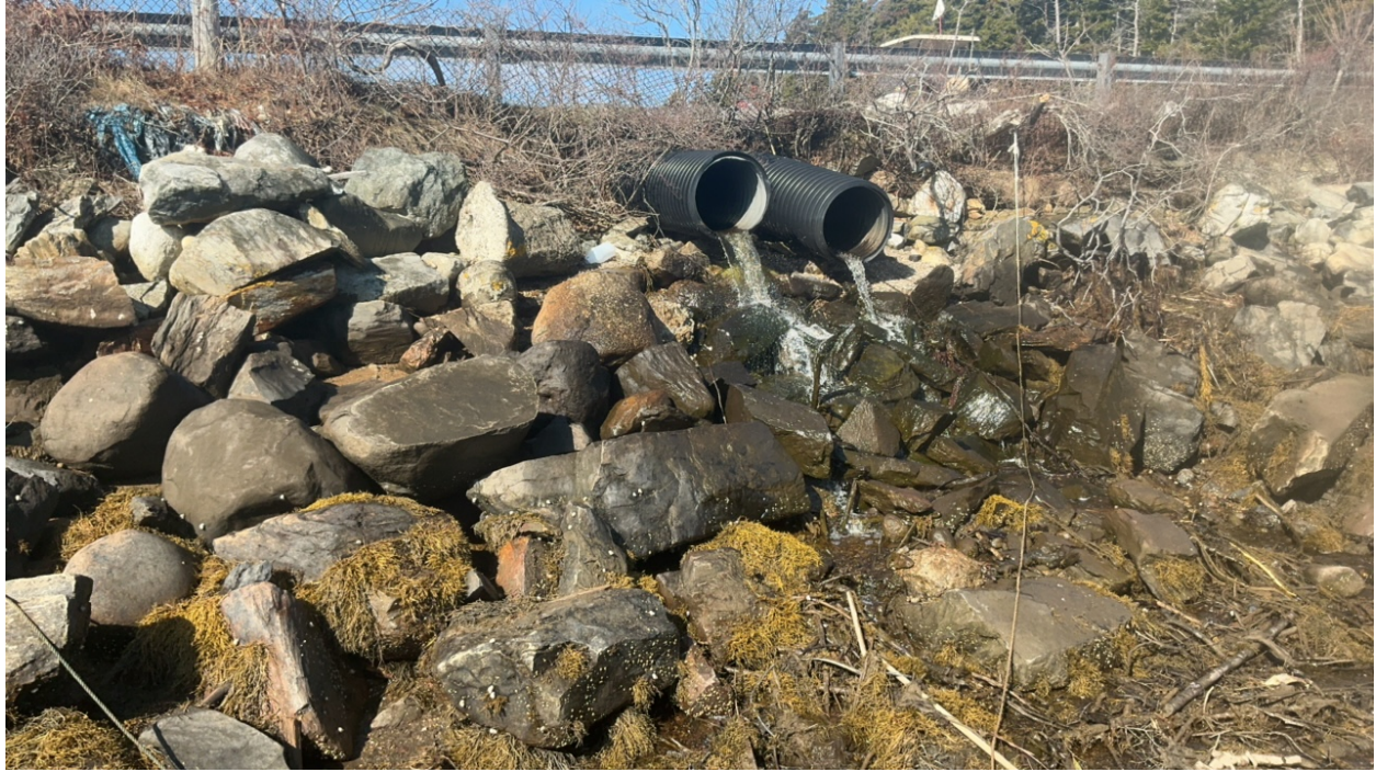
Figure 3: The tidal shoreline adjacent to Fern Avenue and the culvert outlets.
