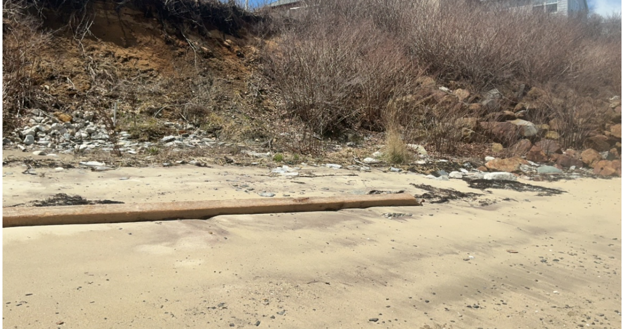
Figure 3: A section of the beach and coastal bluff at the East End site, including the transition to riprap stabilization of the bluff at the neighboring property line.
