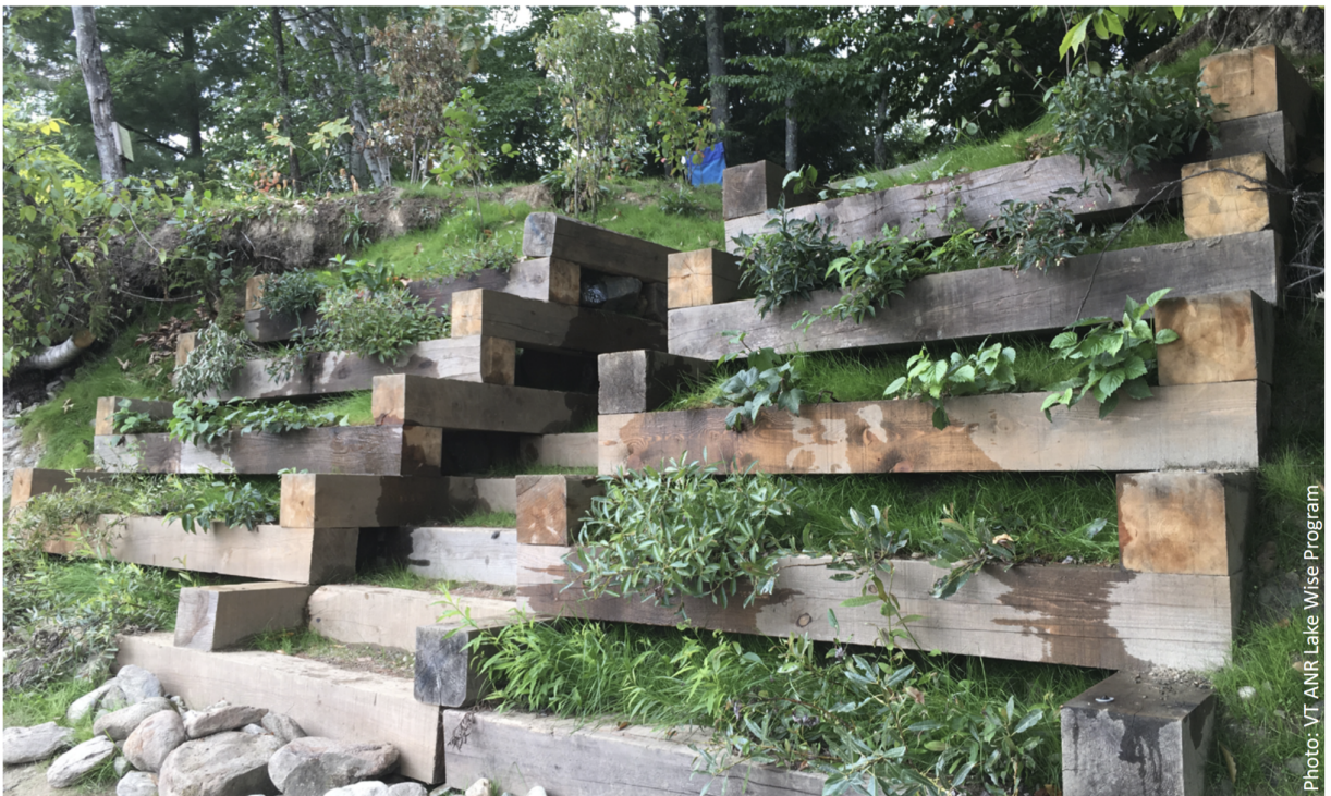
Figure 8: Example of a living crib wall from the Vermont Bioengineering Manual.
