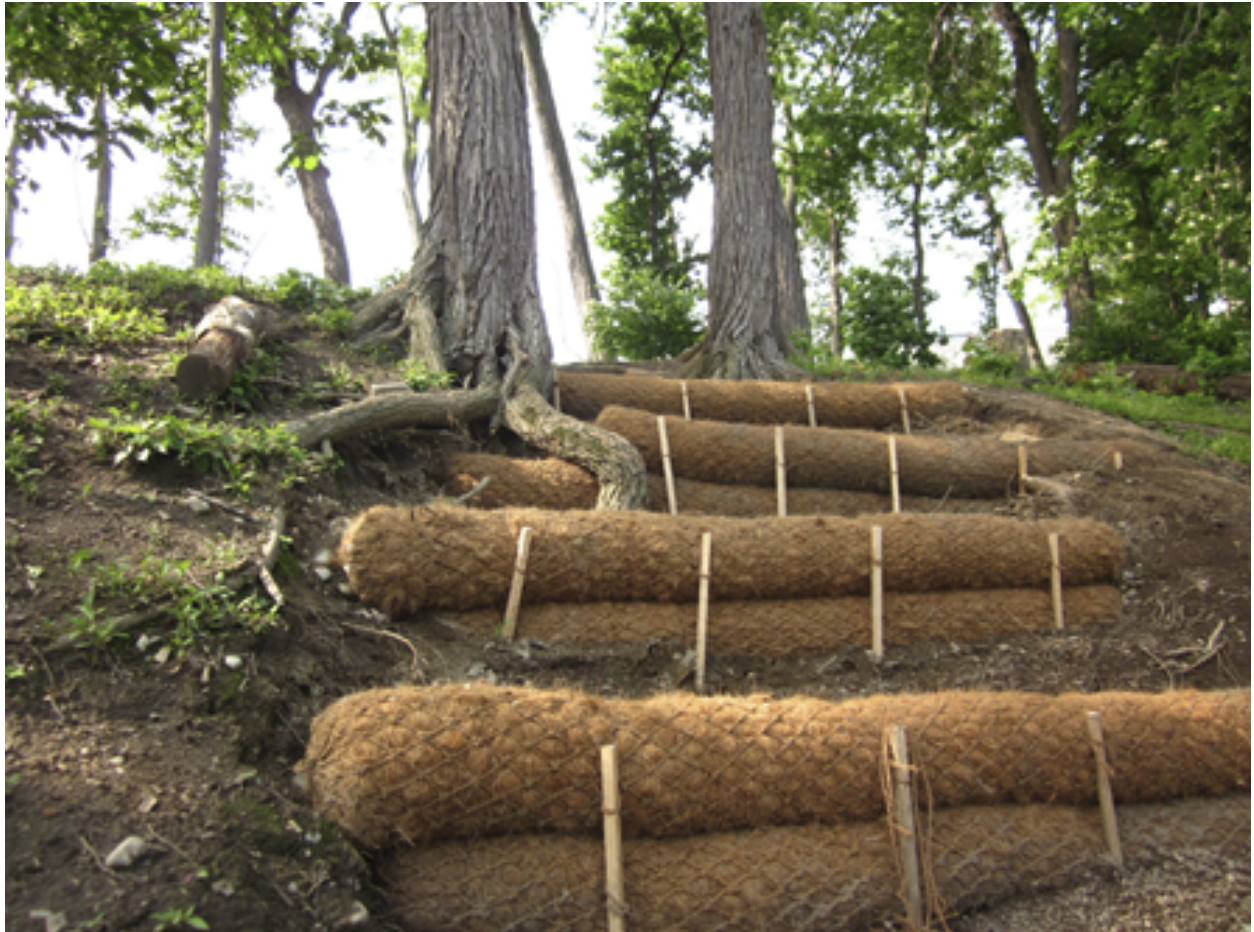
Figure 10: Coir logs used to divert water and repair a gully (Photo from Cambridge Water Department).
