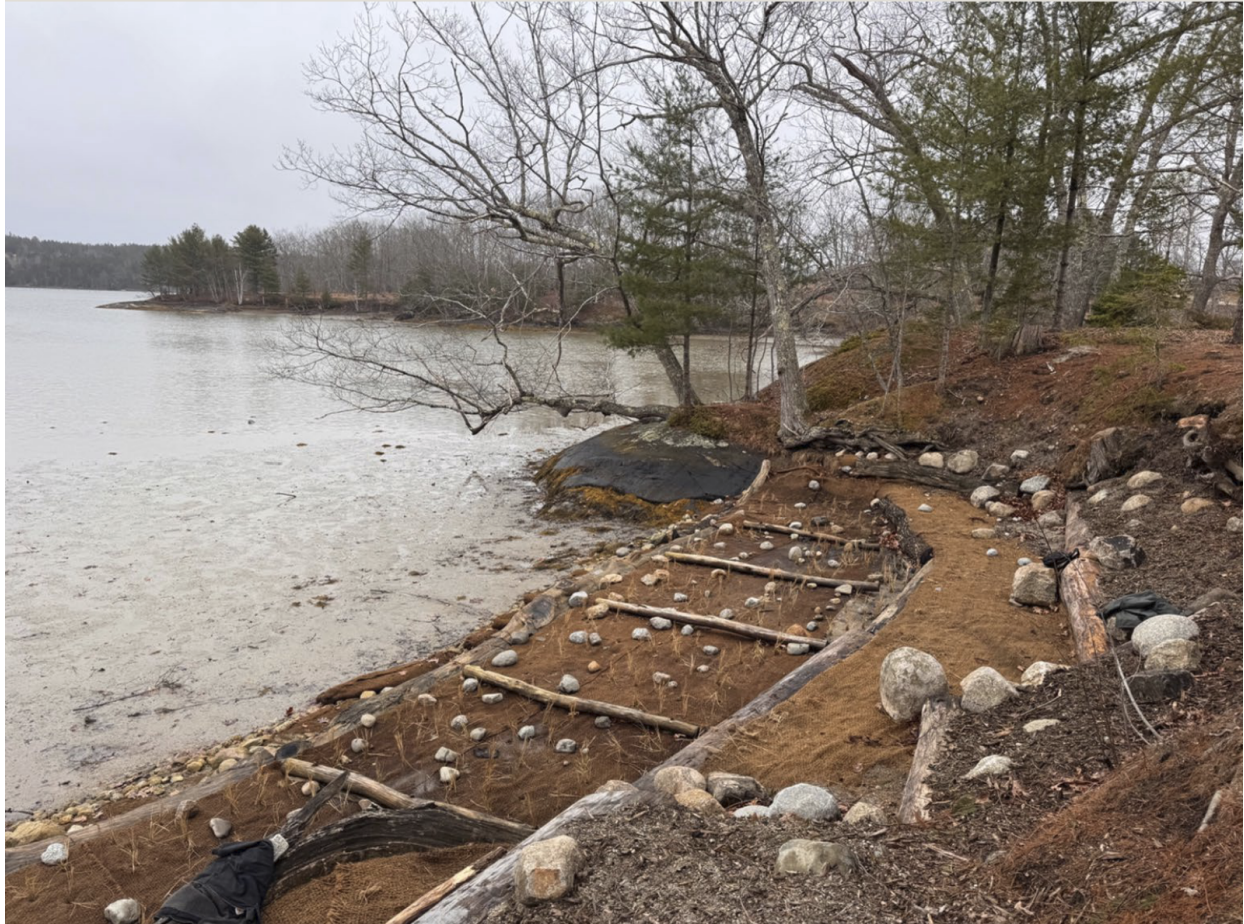
Figure 11: Example of a log sill installed for marsh restoration. (Photo from Treyball & Bernacki, 2025).
