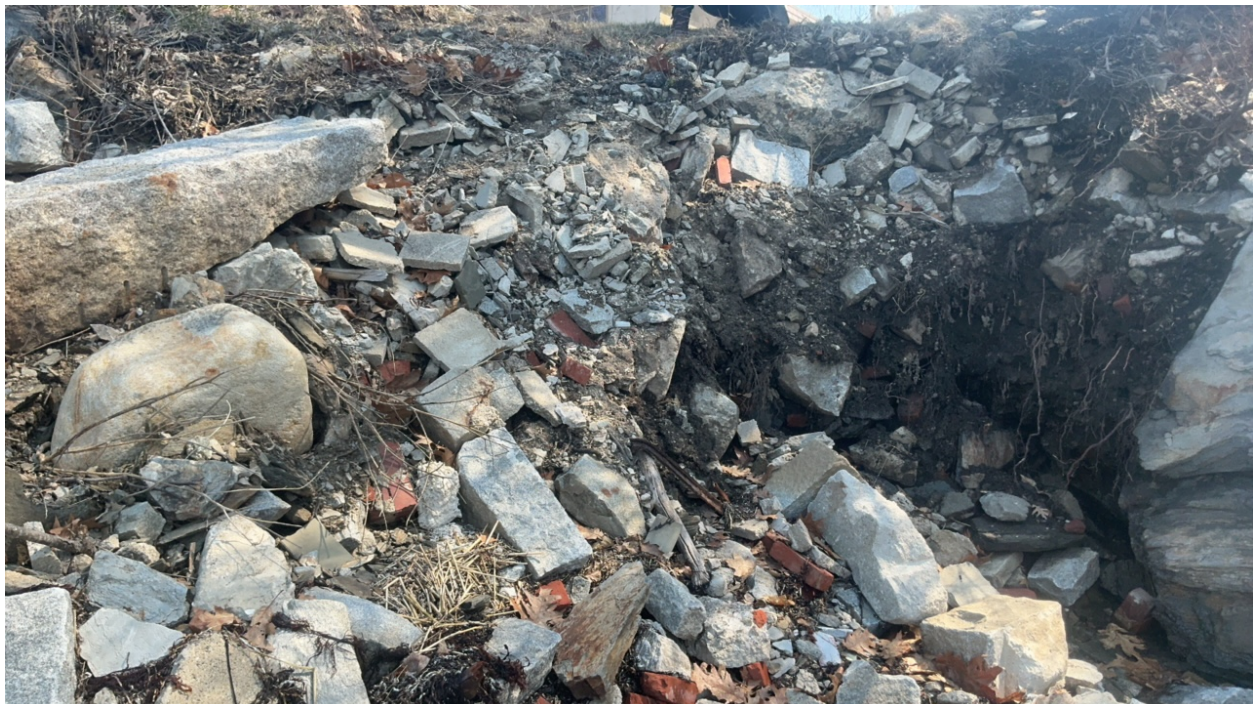
Figure 4: Water now drains from this section of bank after a drainage pipe failed. Bricks and debris are visible in the bank.
