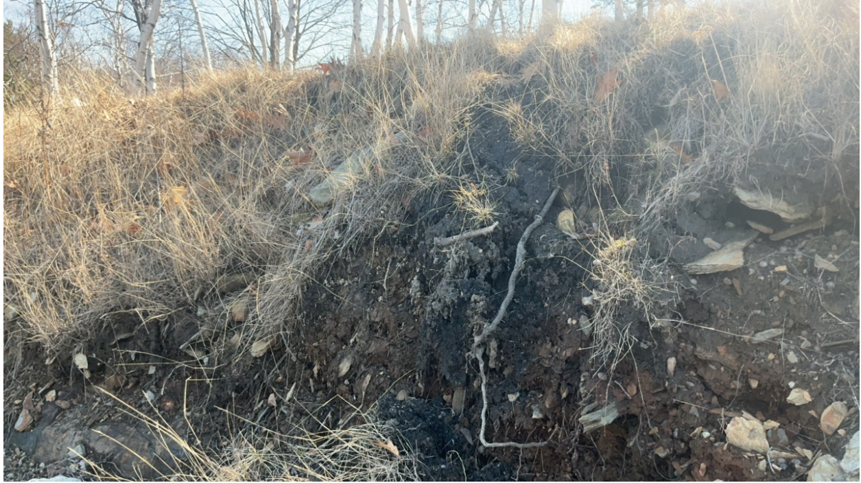
Figure 5: Soil erosion is visible above the top of the placed stone in this section of bank adjacent to the barge landing.
