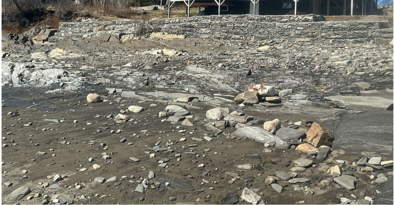
Figure 3: Photograph of the second property including gabions installed for shoreline stabilization.
