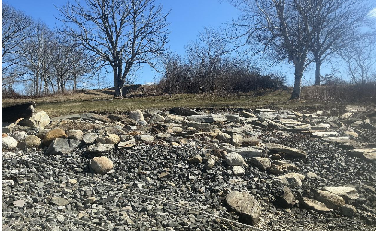
Figure 2: Photograph of the beach and lawn area of Griffin's Cove. Larger stones placed for erosion control are visible along the upper beach edge.
