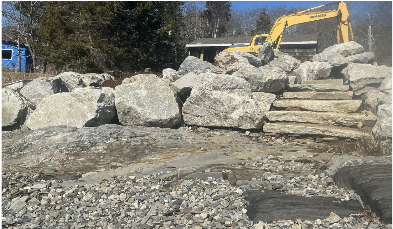
Figures 1 & 2: Photographs of one of two private properties including the stones being installed for shoreline stabilization.
