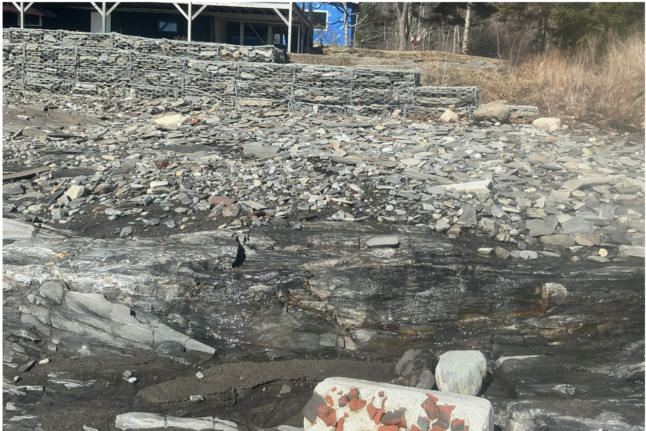
Figure 4: Photograph of the groundwater seep observed on the shoreline.
