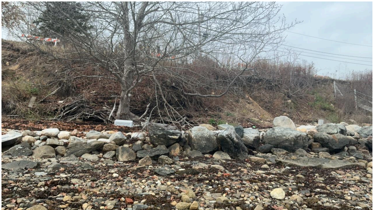
Figures 3 & 4: Photos showing sections of the bluff including access stairs, fallen and leaning trees, and rocks placed in a previous shoreline protection attempt.
