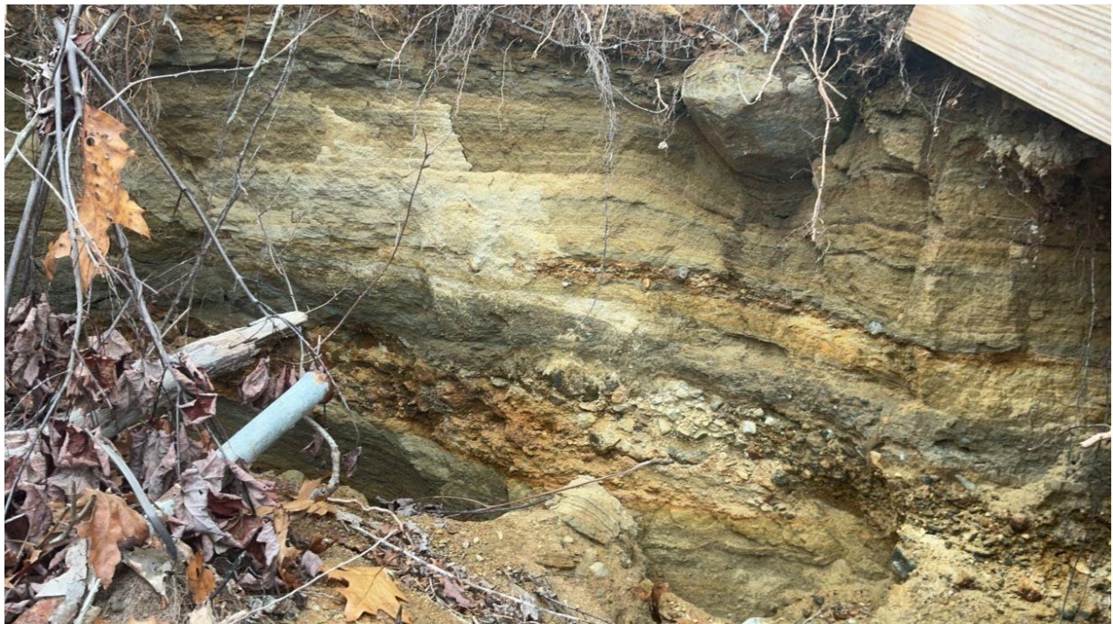
Figure 4: Close-up photo of the bluff sediment taken near the access stairs. Layers of sandy and clay soils are visible.
