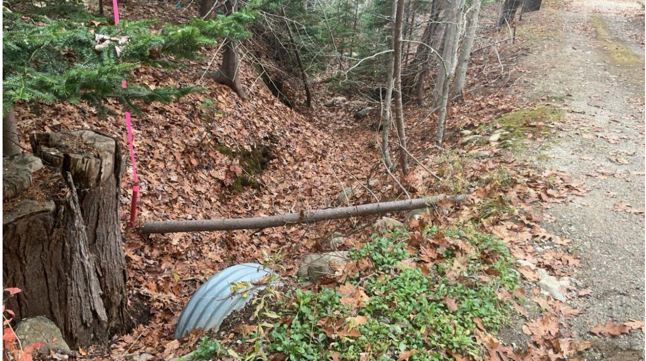
Figure 1: The culvert and seasonal stream located at the north edge of the property.
