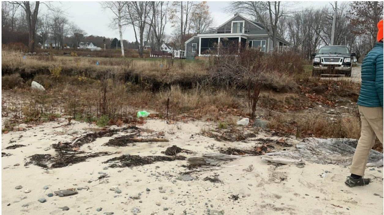
Figure 2: Photo of the Hamilton Beach ROW facing inland.
