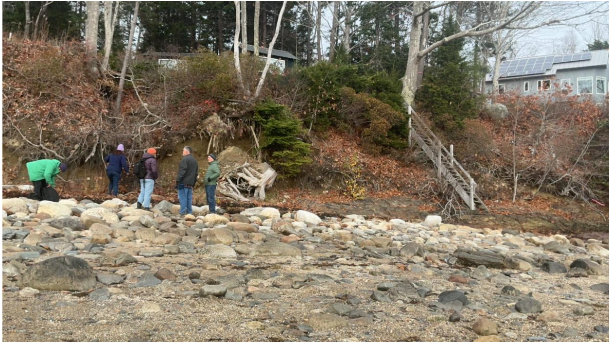
Figure 3: Partial view of the bluff face and intertidal zone. A tree stump that has fallen as a result of erosion and slope failure is visible near the center of the photo.
