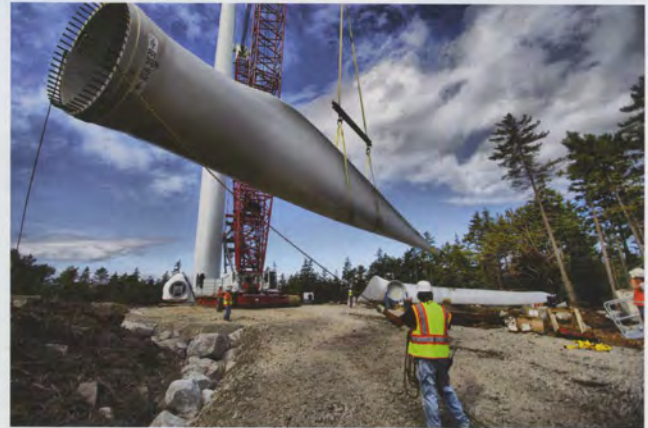
Building the turbines (clockwise from left): Cianbro workers position the nacelle on the top of turbine 1; a turbine hub is hoisted; cranes lift blades; George Baker watches.
