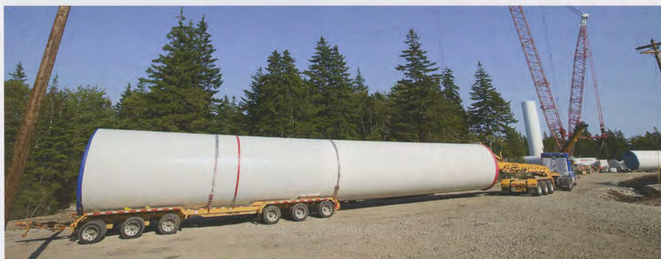
A tower component is delivered to the site.
