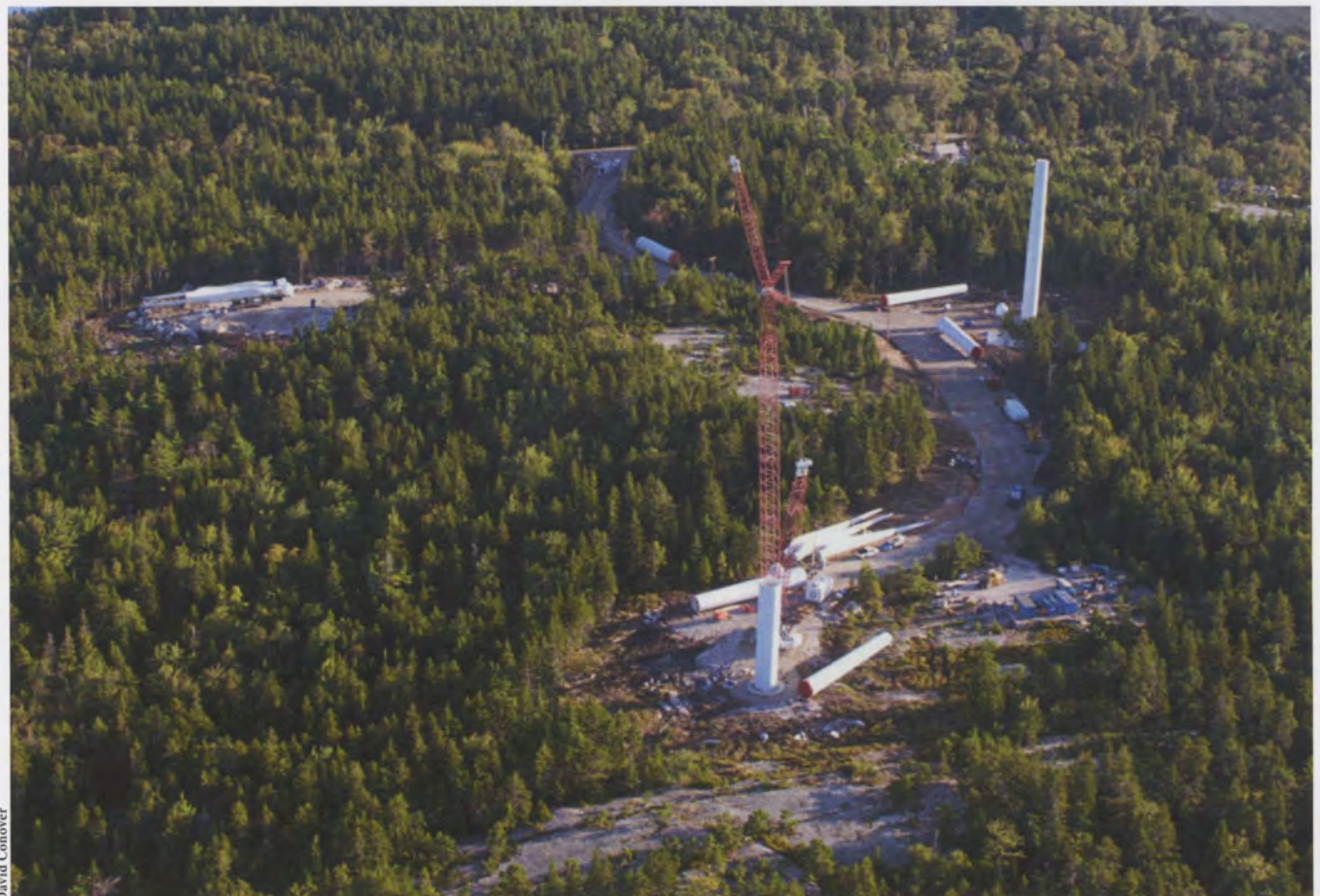
Cianbro workers position the first component of turbine 2.
