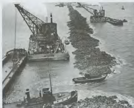
Above: Map of The Netherlands, 1658. Below: Building the Afsluitdijk, which extends from Den Oever in Wieringen to the village of Zurich in Friesland. The dike is about 20 miles long, 300 feet wide and 25 feet above sea level.
