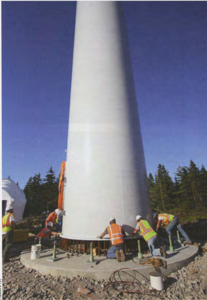
Cianbro workers position the first component of turbine 2.
