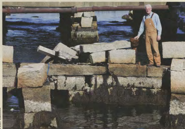
Phil Crossman at the site of the Vinalhaven demonstration project. Crossman and the Ocean Energy Institute are collaborating on a project to rebuild a granite tidal dam that once provided mechanical power for a granite polishing shed. The new dam would produce electricity.
