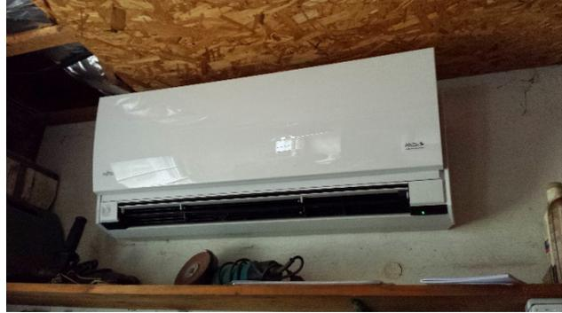
*A ductless mini-split heat pump installed in a lobsterman's workshop on Islesford.*
